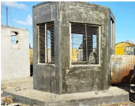
a) El Marsa desalination plant water intake tower
