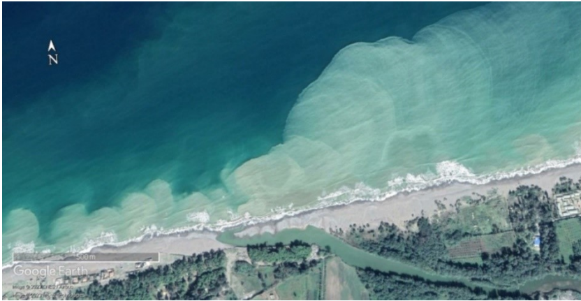
Figure 14: Agrioum River withdrawal for the month of November 2019. Very concentrated suspension evacuated through the dam gates into the sea (Google Earth)
