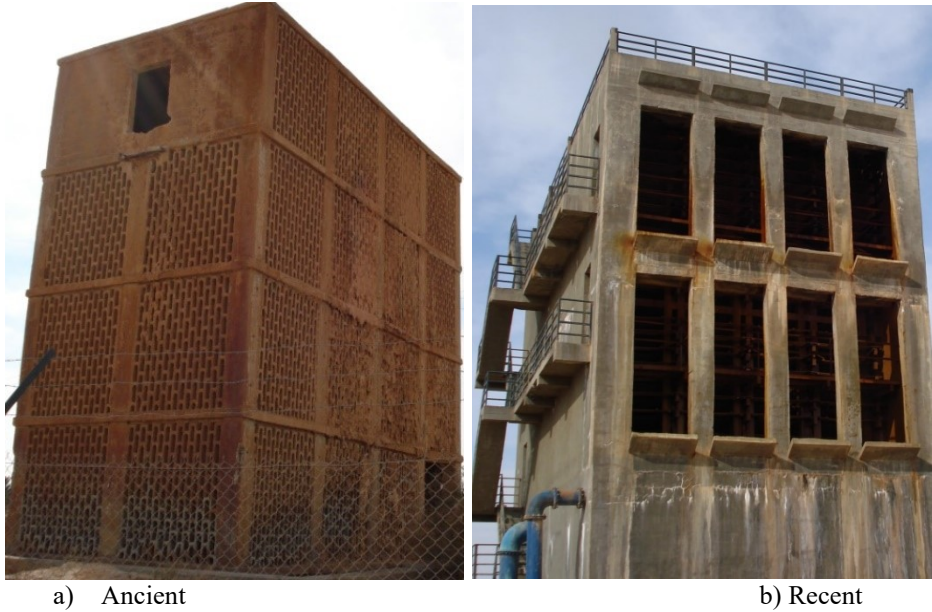
Figure 20: Cooling system for brackish waters of the Northern Sahara aquifer system (Photo. Remini, 2006).
