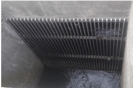
c) Screening of coarse and fine particles from the El Marsa station
