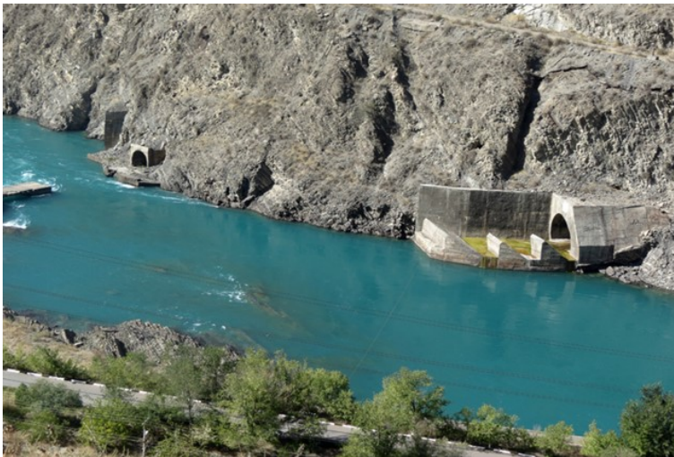
Figure 3: View of the outlet heads of the surface and deep spillways of the Kurpsai HPP + (1976-1986) located in a narrow gorge
