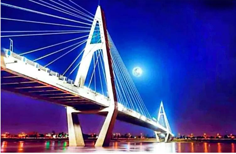
**Figure 1: Ahwaz Eighth Bridge, Iran, supported by inclined piers (Karimi et al., 2017)**
