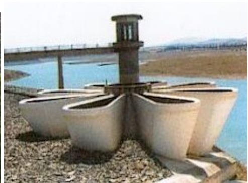
b) Tulip-type flood spillway (Photo. Remini, 2006)
