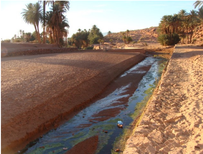
c) After passing a flood, the Tiout Dam finds itself silted up again with the same quantity of mud removed (Remini, 2022)
