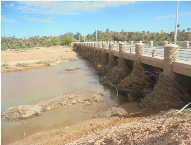
Figure 15: The bridge piers on Wadi of Saoura favored the formation of a temporary dam made of brush and palm tree trunks. The latter gave way to the pressure generated by the rapid rise of the water. This is the hammer blow of the Saharan flood. (Photo. Rezoug, 2014).
