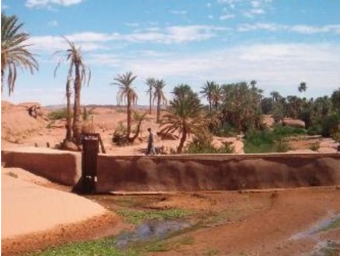
Figure 12: Tiout River – Flood of May 30, 2020. The ancestral dam is no longer. The hydrotechnical heritage was washed away by the Saharan flood (Photo. Remini, 2009).
