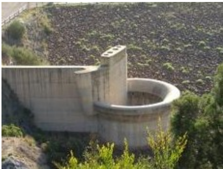
b) Tulip-type flood spillway (Photo. Remini, 2006)
