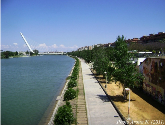
Figure 4: Guadalquivir riverbank development- City of Sevilla (the author, 2011)
