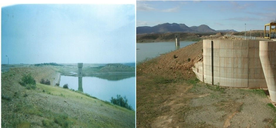
Photograph 1: General view of the Ouizert Dam – Algeria (Benfetta, 2018).
