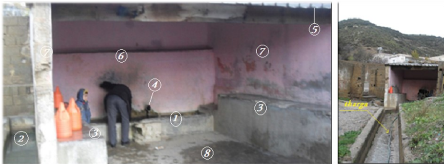
Photo A : 1-inner pool 2-watering trough 3- akdane 4-asherchour 5- roof in metal sheeting 6- "asherchur" wall 7- lateral wall 8-the floor of thala Photo B : Tharga
