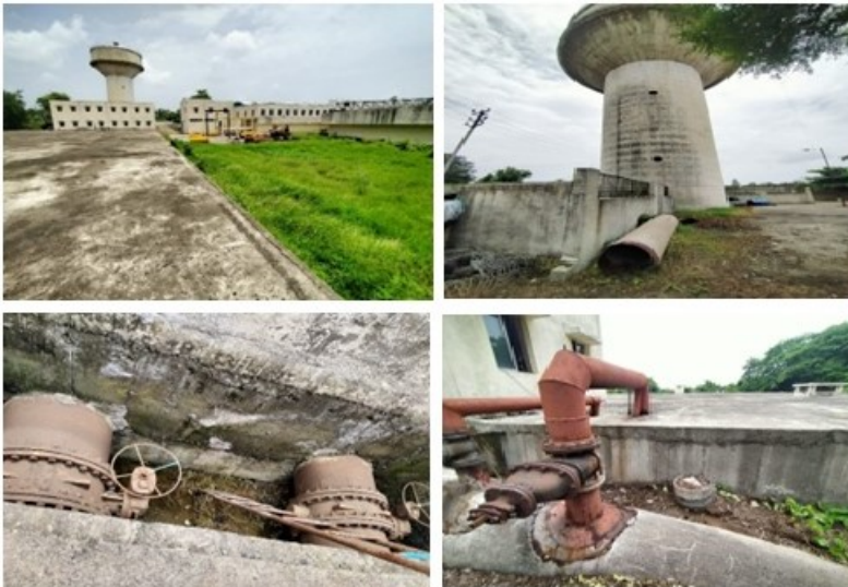
Figure 2: Site Visit at Variav Headwork, Surat City
