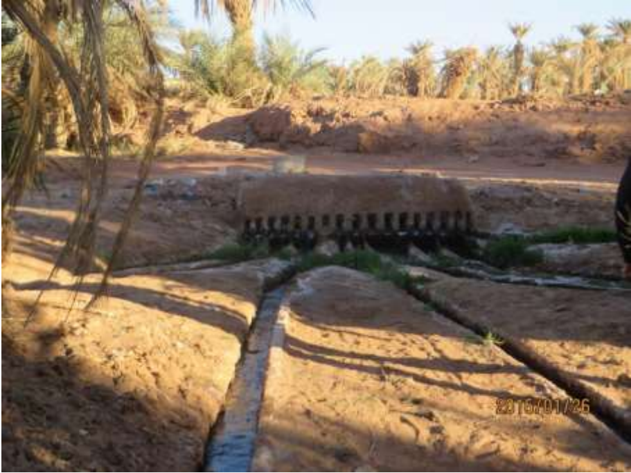
Figure 28: Secondary Kasria of the foggara of El Meghier of the Timimoun oasis (Photo. Remini, 2015)
