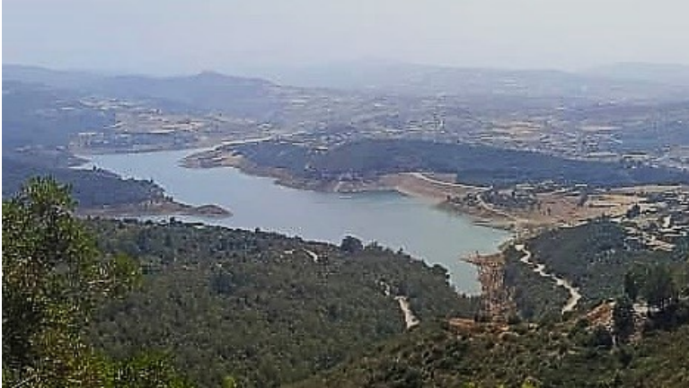
Figure 4: Keddara Dam, the water tower of Greater Algiers during the 1980s and 1990s, suffered two water shortages during the period 2000-2024 (Photo from Remini, 2024).
