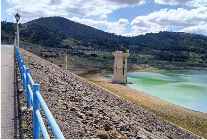
Figure 5: Boukourdane Dam in a critical situation. Due to a low siltation rate, the dam exploits the waters of the dead volume to satisfy its demand for drinking water (Photo from Remini, 2024).
