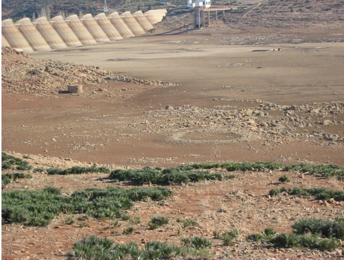
Figure 3: Mefrouch Dam, Drying of the dam lake following the phenomenon of evaporation; Image that will be repeated in the coming years (Photo from Habi, 2006)
