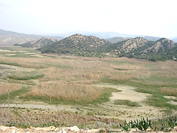
Figure 5: Fergoug Dam Lake filled with mud. Dam silted up to 85% of its initial capacity (Photo Remini)
