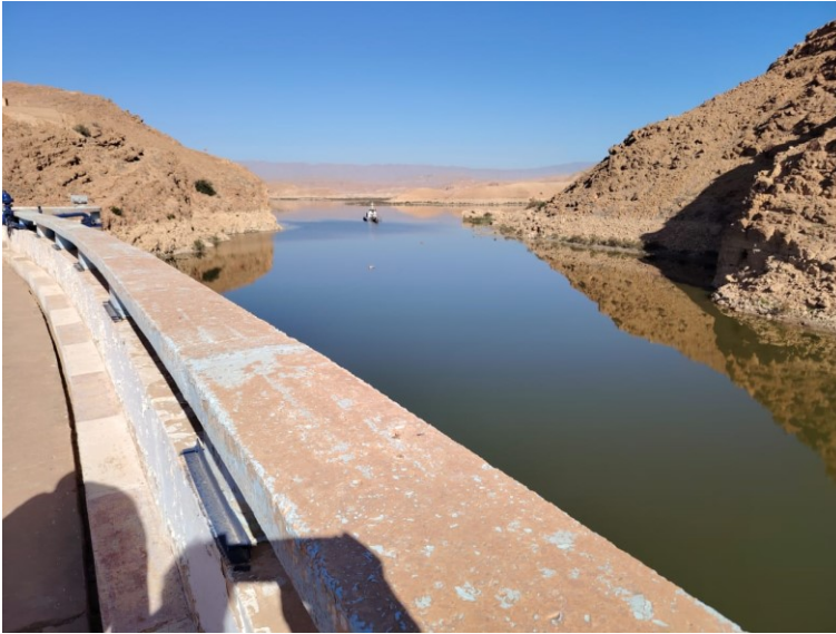
Figure 2: Foug El Gherza Dam. Dam silted up and dried up? For 6 years, the water level of the dam has been at dead volume (Photo Remini, 2024)
