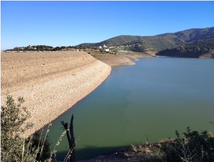
Figure 1: Keddara Dam. Dam not silted up but dried up? During the period 2000-2024, the level of the dam reaches 3 times the dead volume (Photo Remini, 2024)
