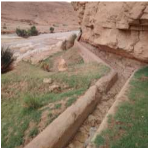
Figure 27: Seguia Gharbia in the River Labiod. After an irrigation operation by flooding the entire palm grove with flood waters, the seguia must be cleaned of sediment deposits (Photo. Remini, 2025)
