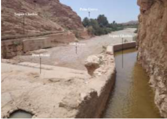
Figure 36: The parallel seguias of the Branis dam on Wadi Abdi (Photo. Remini, 2025)
