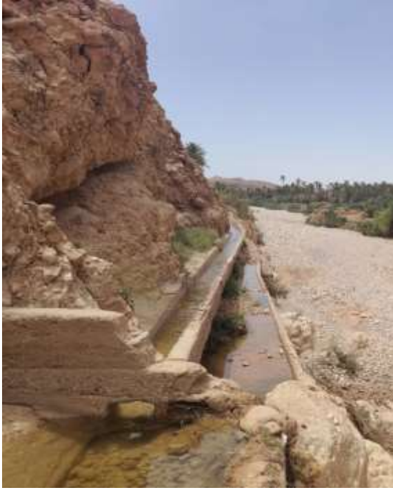
Figure 28: Two superimposed seguias emanating from the Branis dam on the Abdi wadi (Photo. Remini, 2025)
