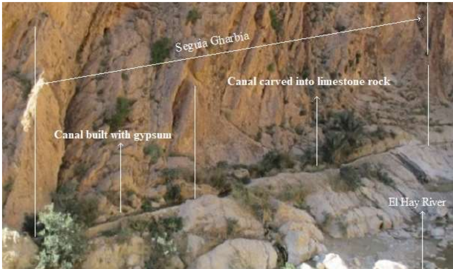
Figure 29: The section of a section of a Gharbi seguia emanating from the dam on the El Hay wadi was carved into the limestone rock (Photo. Remini, 2010)
