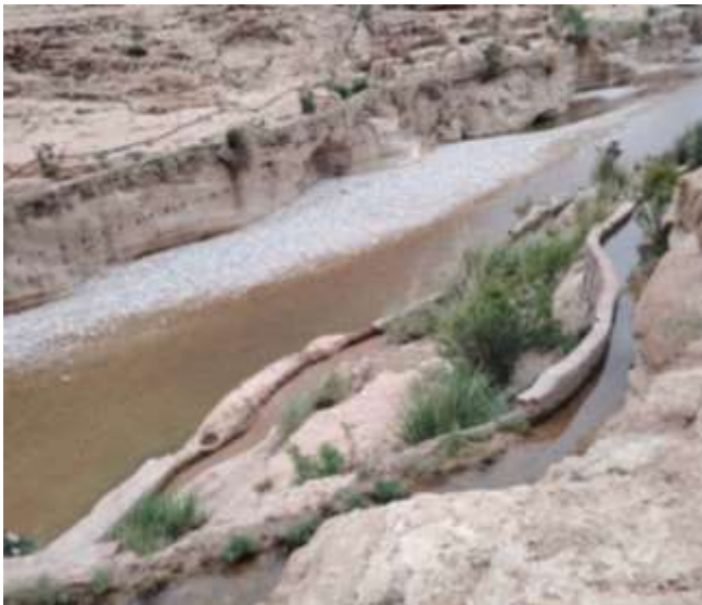
Figure 34: A system of 3 seguias emanating from the system of two Mchounech dams on the River Labiod (Photo. Remini, 2025)
