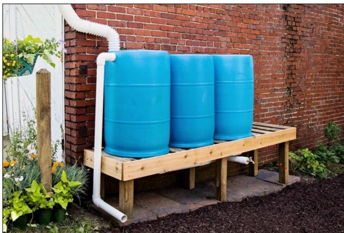
Figure 3: Barrel rainwater harvesting (Peters, 2016)
