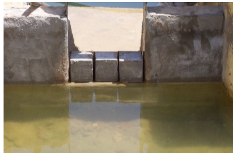
Figure 2: Schematic Illustration of a Concrete Fuse plug
