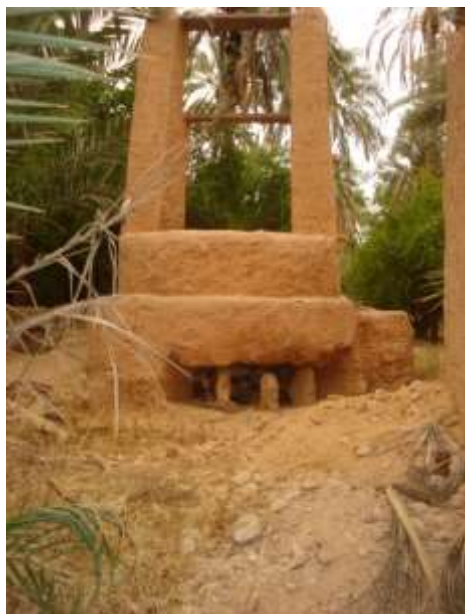
Figure 38: Recharge well in the Ghardaïa oasis equipped with an opening to allow floodwater to fill the well (Photo. Remini, 2012)
