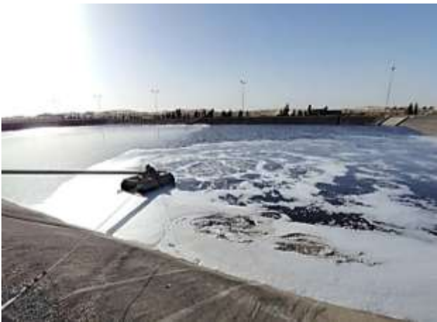
Figure 15: Souf valley Lagoon Wastewater Treatment Plant (Photo. Remini, 2024)
