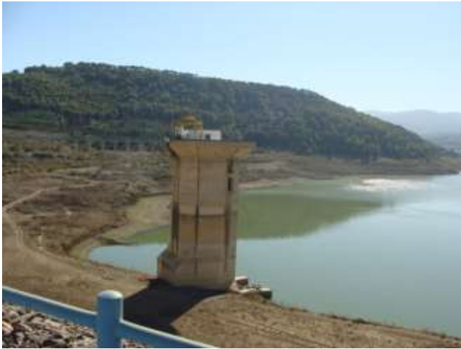
Figure 3: Boukourdane dam. For the second year, the dam is using its dead volume (Photo. Remini, 2025)
