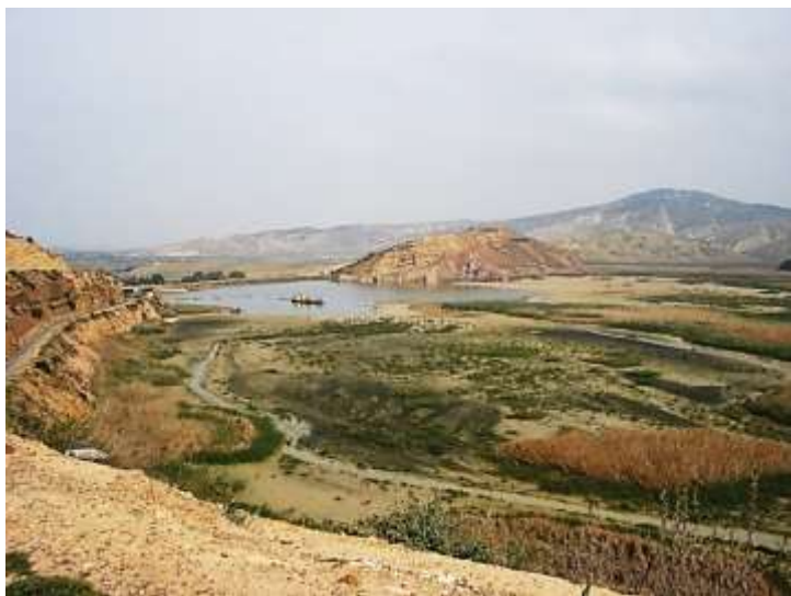
Figure 11: Fergoug Dam silted up to more than 90% of its capacity (Photo. Remini, 2009)
