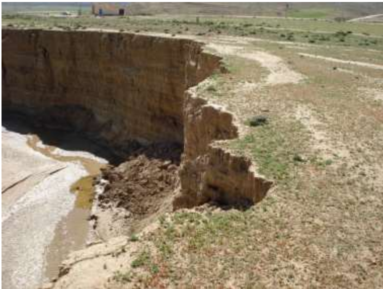
Figure 8: In recent years, the Chelif River has widened (Photo. Remini, 2013)
