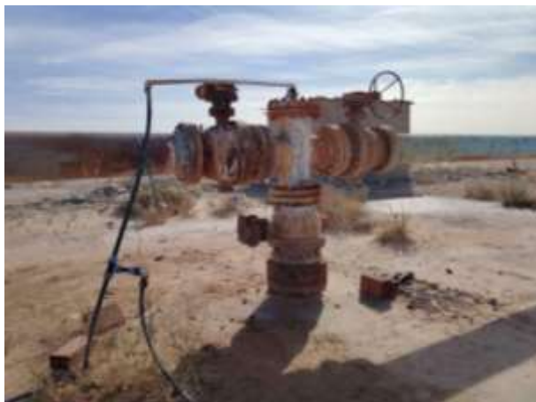
Figure 14: Touggourt, Albian borehole over 1800 m deep (Photo. Remini, 2023).
