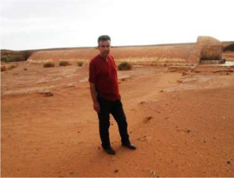
Figure 28: An overview of the covered dam in the El Guerrara region (Photo. Remini, 2009)
