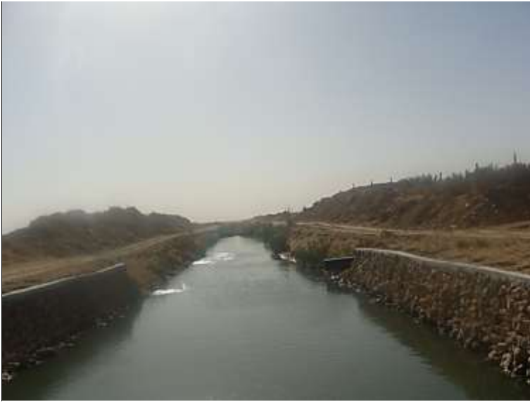
Figure 16: Canal carrying drainage water from the palm groves of Touggourt (Photo. Remini, 2023)
