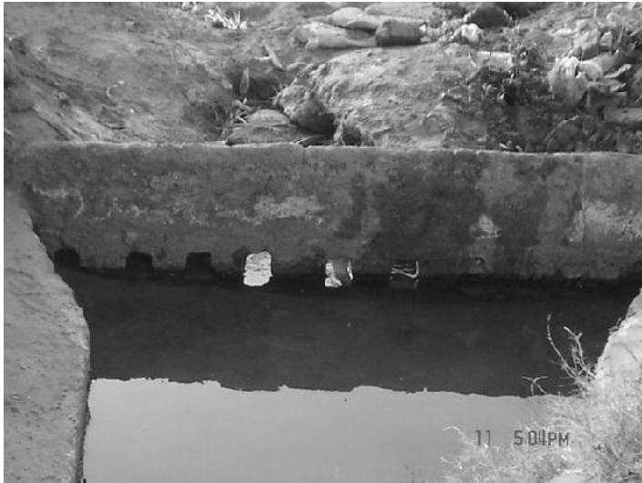
Figure 5 : Kasia of the foggaras of Ezzoua (In Salah)
