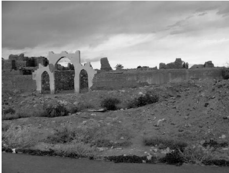
Figure 8 : Overview of Ksar Kenadsa
