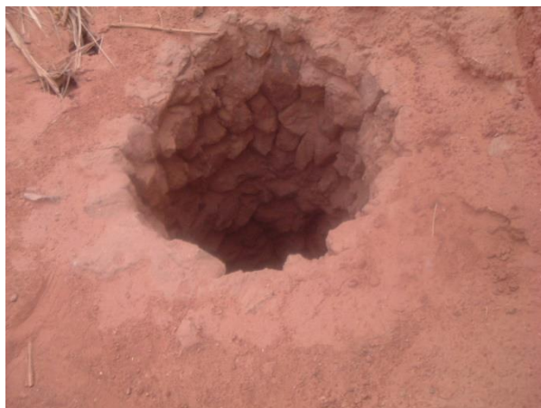
Figure 4 : Air Shaft of Albian foggara (Remini, 2007)
