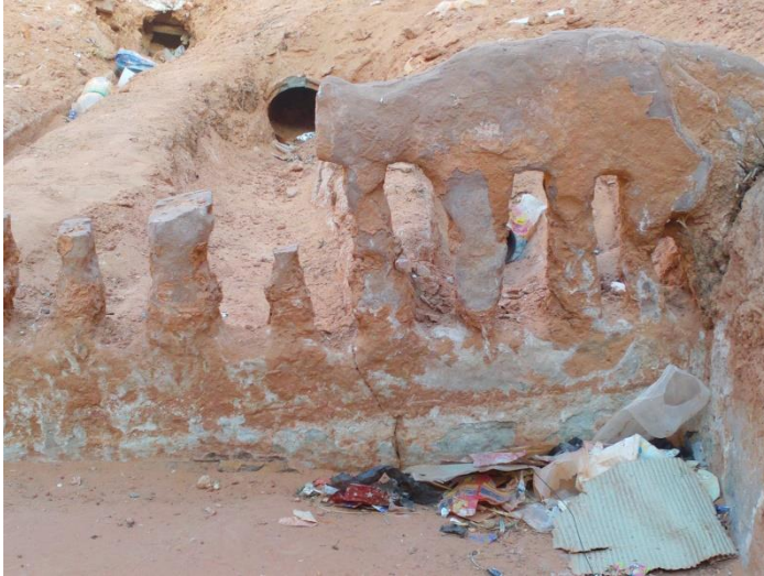
Figure 11 : Kasria of Albian foggara destroyed ( Nouh et Remini, 2010)
