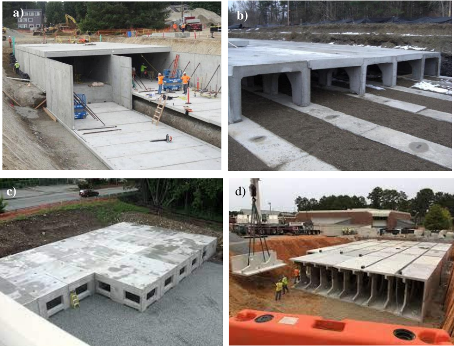
Figure 1: Precast-concrete permeable pavements in the forms of a) panel ( https://oldcastleinfrastructure.com ), b) arc ( https://www.kistner.com/ ), c) box ( https://precast.org/ ) and d) modular unit ( https://stormtrap.com )
