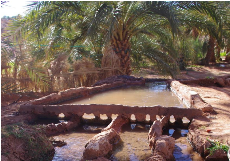
Figure 28: Kasria lakbira of a triangular-shaped foggara of the oasis of Guentour (Photo. Remini, 2019)
