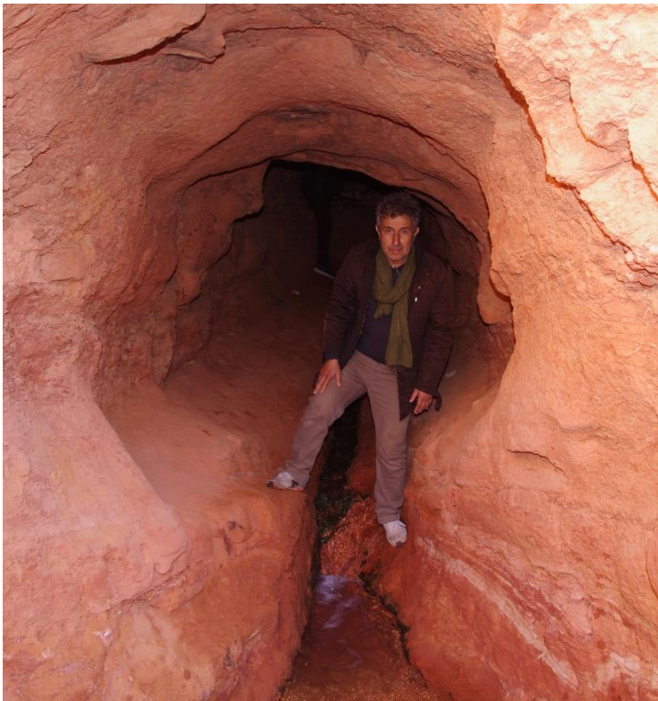
Figure 25: Transport part of the gallery of foggara of the Timimoun Oasis (Photo. Remini, 2019)
