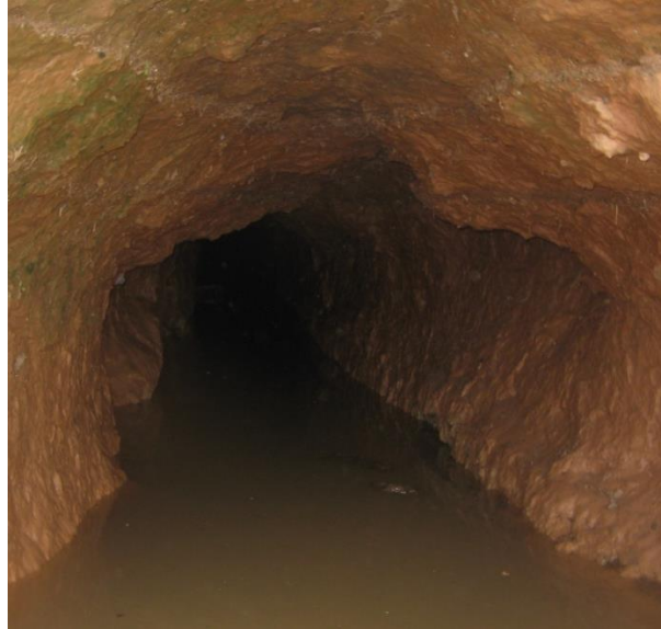
Figure 18: Draining part of the Tindouf foggara gallery (Remini and Abidi, 2019)
