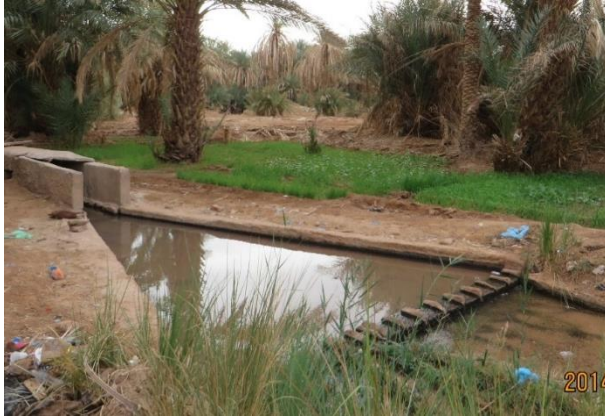
a) Mega kasria of a foggara in the Augrout oasis (Photo. Remini, 2014)
