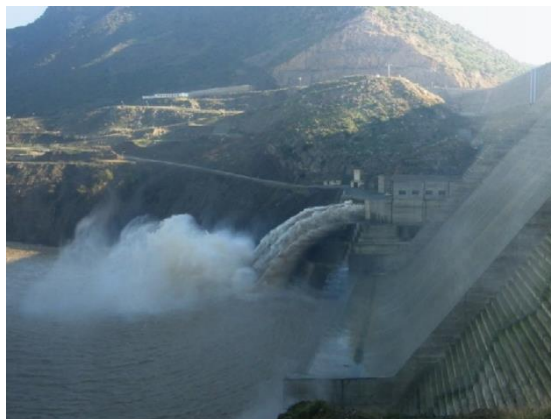
Figure 9: Withdrawal Operation of Dams. (photo. National Agency for Dams and Transfers)
