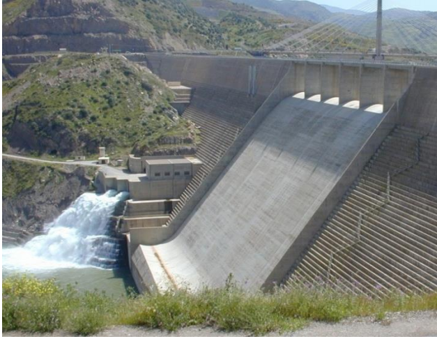
Figure 10: Withdrawal clear waters; synonym of the end of density currents (photo. National Agency for Dams and Transfers)
