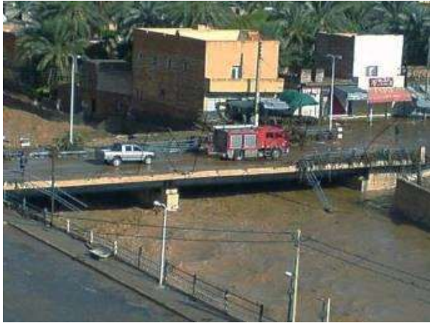
Figure 3 : L'oued Metlili en crue (Crue 12-13 /03/2011 Debit max = 570m 3 /s) (Photo. Ouled Belkhir, 2011)
