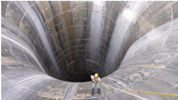
Photo 1 : Shaft spillway- vertical shaft with funnel-Shaped mouth
