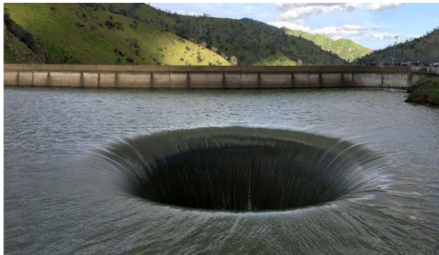
Photo 2 : Shaft spillway in operation under small head over the crest
