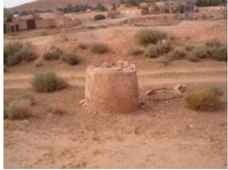
b) Tunnel ventilation wells evacuation (Photo. Remini, 2011)
