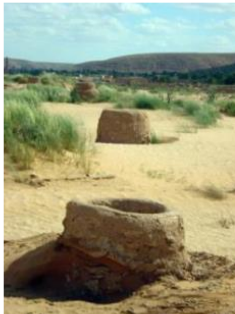
Figure 29: First part of Tardja N'Tkdimt: a Tissanbadh a 180 m gallery equipped with 9 ventilation shafts (Photo. Remini, 2013)
