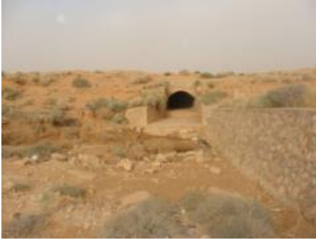
a) Exit from the tunnel to M'zab River (Photo. Remini, 2011)
