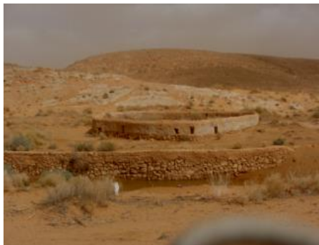
a) Diversion structure
