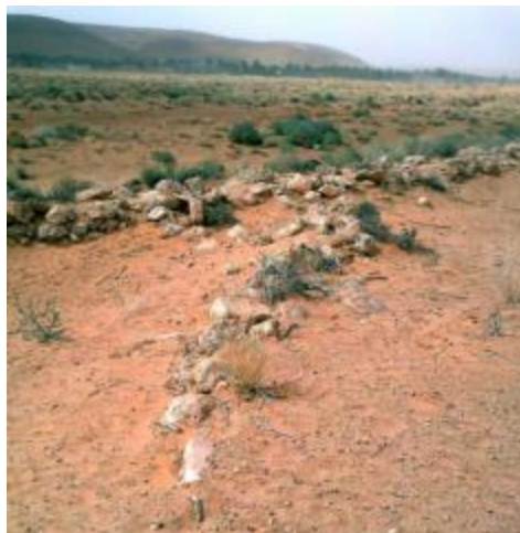
Figure 18: A rip-rap obstacle in the system of deposit thresholds achieved without Tardja N'Bouchemdjane (Photo. Remini, 2008)
