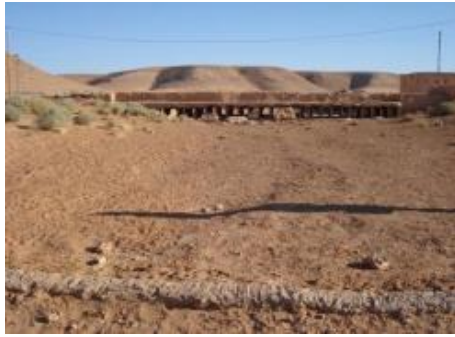
a) Upstream view
