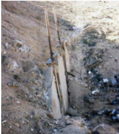
Figure 33: Sliding valves in the second gallery (Photo. Remini, 1998)
