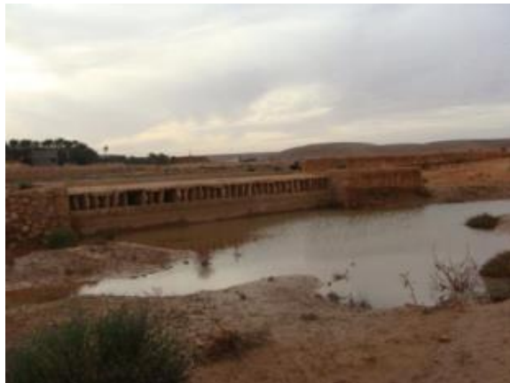
Figure 44: Spillway from the Bouchen dam (Photo. Remini, 2013)
