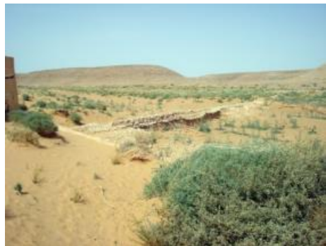
Figure 26: Second Dam - Part of the dike (Photo. Remini, 2013)
