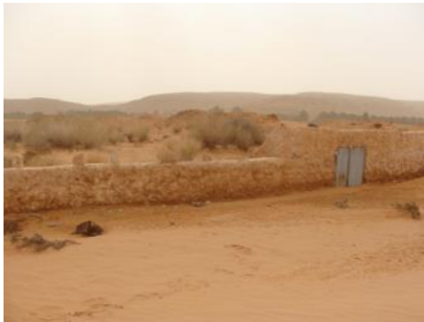
Figure 14: One of the 4 spillways of the Inerz system (Photo. Remini, 2008)
