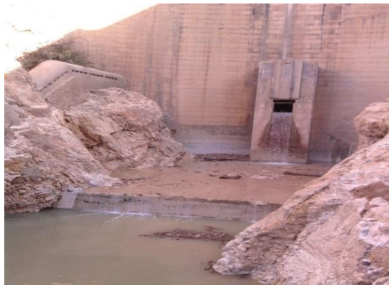
Figure 10: Extraction of sediments in the Foug El Gherza dam By bottom drain (Photo. ANBT-Foug El Gherza Dam)
