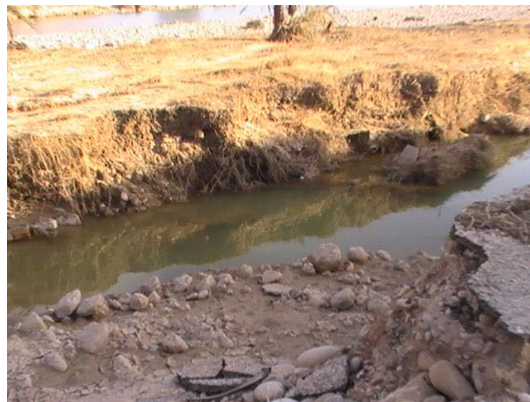
Figure 3: Soil degradation downstream of the watershed (Photo. ANBT-Foum El Gherza Dam)
