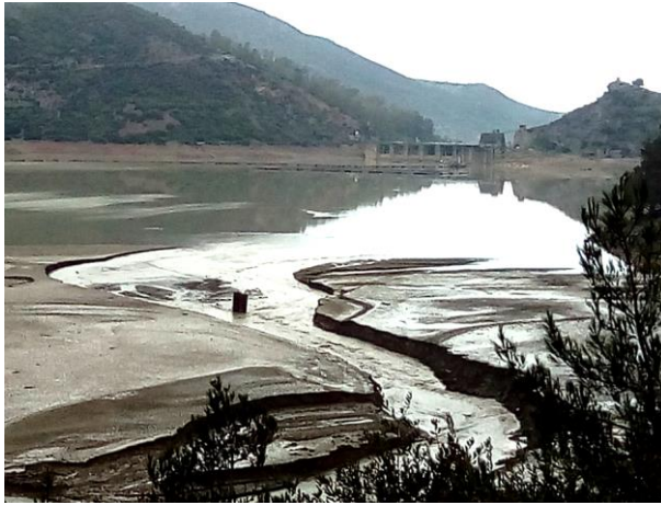
Figure 11: State of the siltation of the Zardezas dam (Photo Toumi, January 25, 2017)
