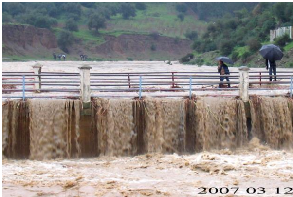
Figure 5: Downstream of the Zerdezas dam. Flood of March 12 and 13, 2007 with a maximum flow rate of 180 m 3 /s (Photo. National Dams Agency, March 12, 2007)
