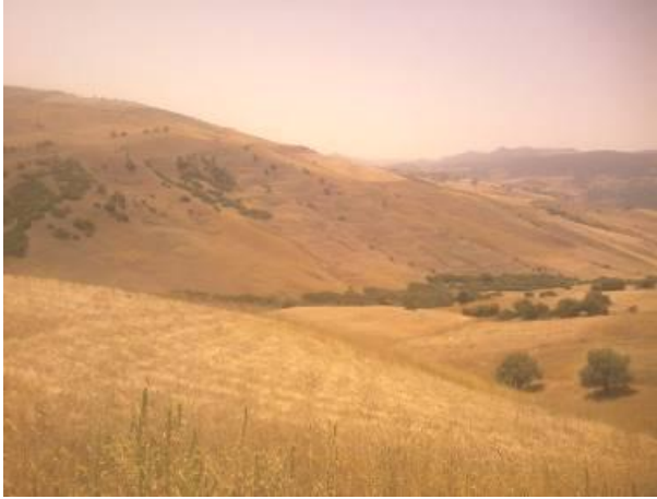
Figure 6: Sheet slide in the slope of the dam des Zardezas (Photo. Toumi, July 8, 2015)
