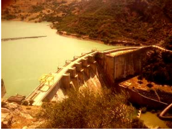
Figure 2: General view of the Zardezas dam (Photo. Toumi, July 2015)
