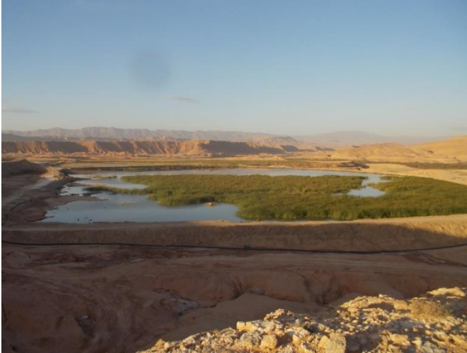
Figure 18: Storage basin for the silt released by the dredging technique during the clearing of the Foug El Gherza dam (Photo. Remini, 2017)
