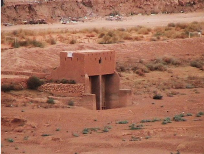
a) Drainage gates to the M'zab River (photo. Remini, 2012)
