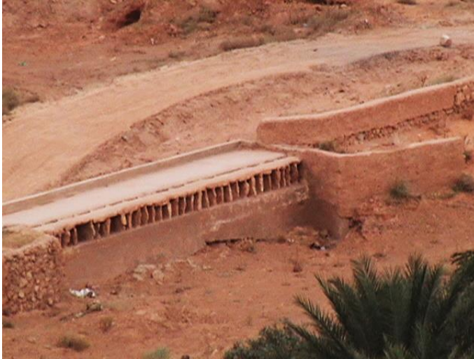
b) Internal face (towards the Bouchen reservoir) (Photo. Remini, 2013)
