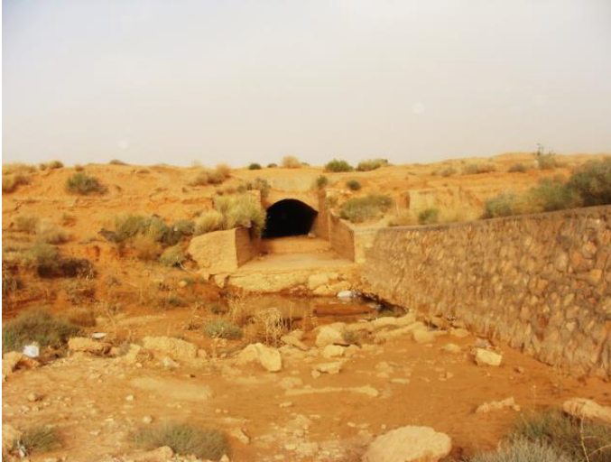
c) Exit from the tunnel to the M'zab River (Photo. Remini, 2011)
