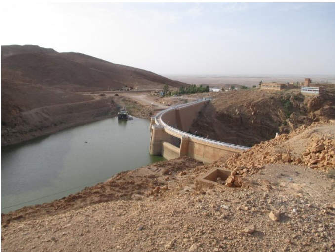
Figure 16: The Foum El Gherza dam silted up at more than 65% of its initial capacity is in the depletion phase (Photo. Remini, 2016)
