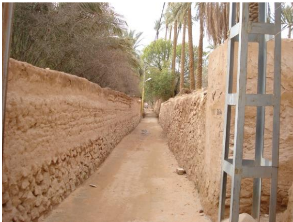
Figure 15: Garden walls built with riprap (foundations) and the upper part (about 3 m) in the ground (Ahbas N'Boucen vase) (Photo. Remini, 2012)
