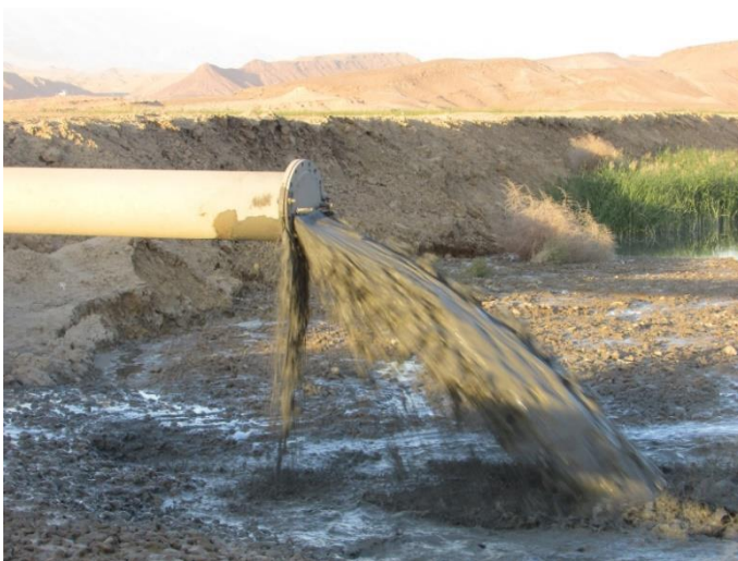
Figure 17: Release of silt into a storage basin during dredging of the Foum El Gherza dam (Photo. Remini, 2017)
