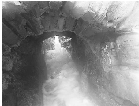
c) Water outlet from the mill
