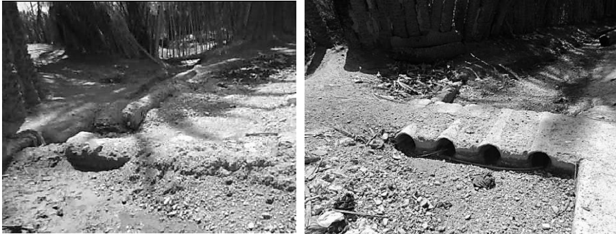
Figure 19: Deteriorated and abandoned Souagui (Photo. Remini and Hareche, 2016)
