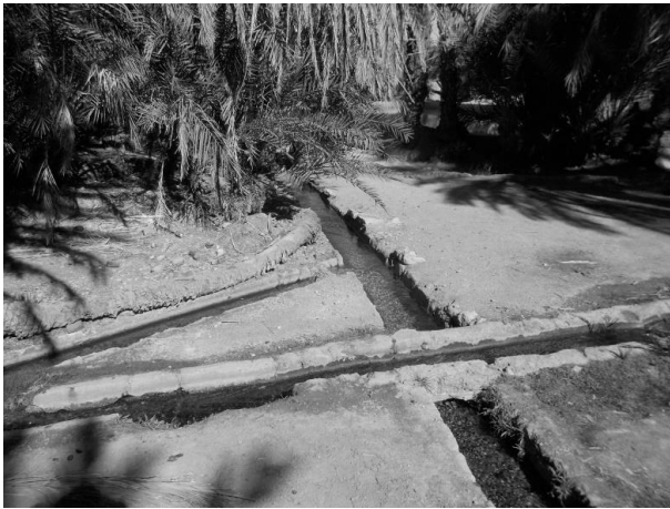
Figure 14: A water distribution network without the Kasriates in the Boukais palm grove in the Saoura valley (Photo. Remini, 2014)
