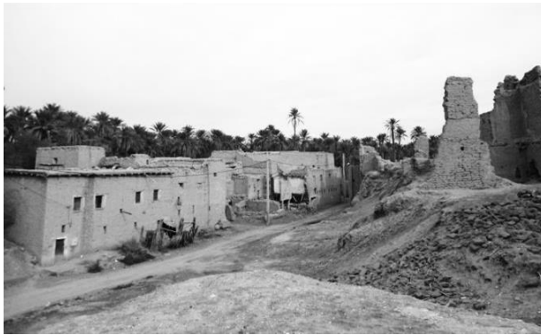
Figure 2: A view of the Dechra of Chetma (Photo. Remini and Hereche, 2016)
