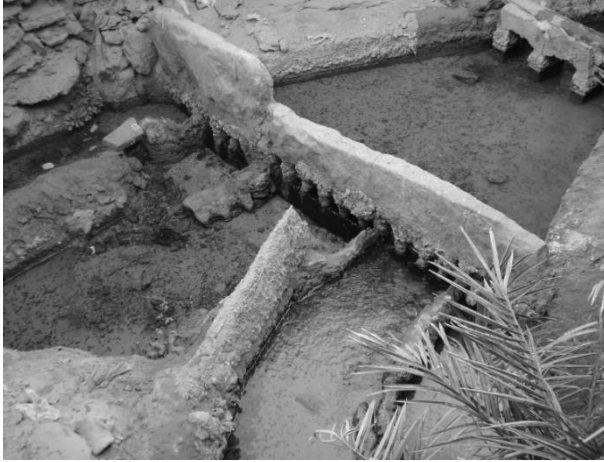
Figure 13: Kasria Lakbira of the foggara Meghier in the oasis by Timimoun (Photo. Remini, 2008)
