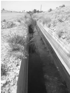
a) Canal on the ground (Photo. Remini, 2017)
