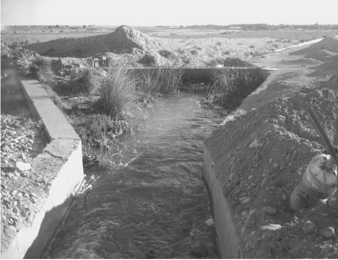
Figure 20. Even the first Mekssem at the arrival of the main seguia takes the form of a triangular basin like that of the kasria (Photo. Remini, 2012)
