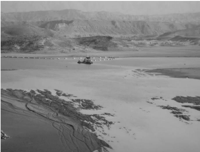
Figure 13: A view of the siltation condition of the Foug El Gharza dam (Photo. Remini, 2018)
