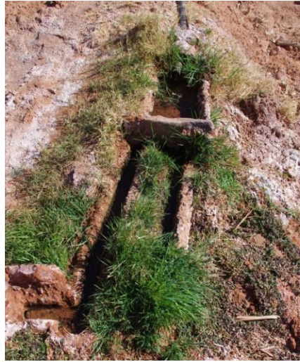
Figure 7: Tertiary Kasria from a Foggara in the Tidikelt (Authors, 2013)
