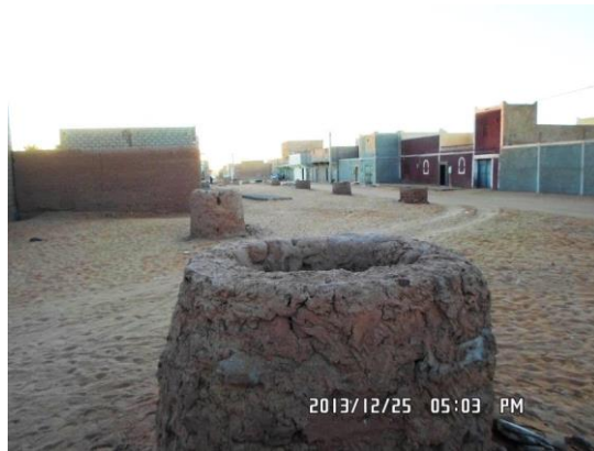
Figure 4: Ventilation wells of a Foggara in Tidikelt (Authors, 2013)
