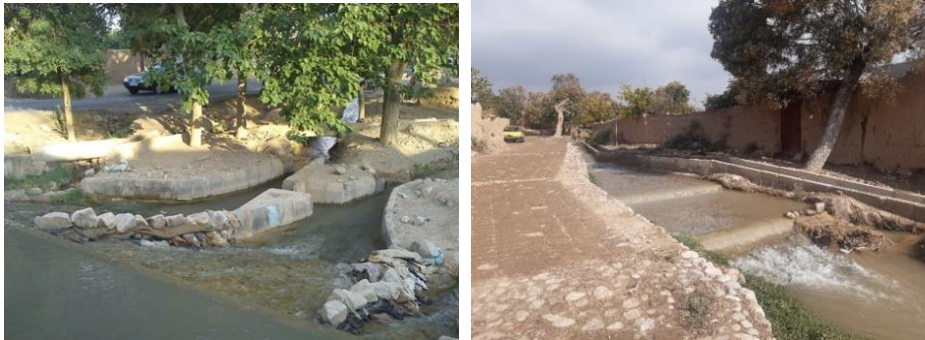
Figure 8: Examples of secondary water dividers in main streams among the orchards. Photos by: left: M.Jamshidian, 2011 & right: S. Lavaf, 2020.
