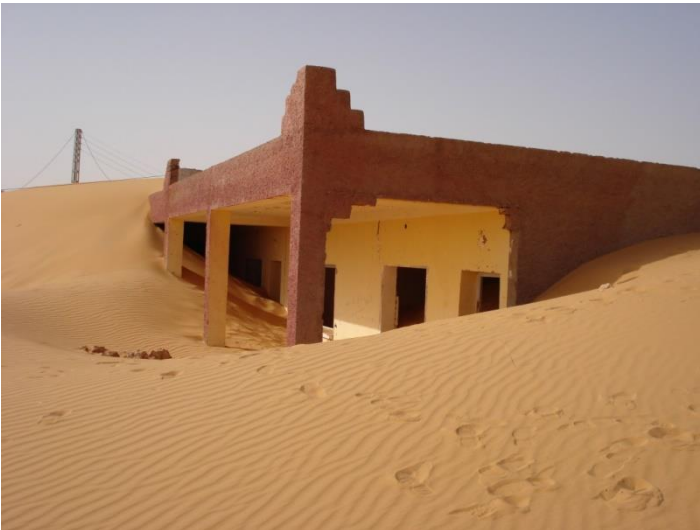
Photo 4: A school in the oasis of Timimoun is under the sand from the Grand Erg Occidental (Remini, 2008)
