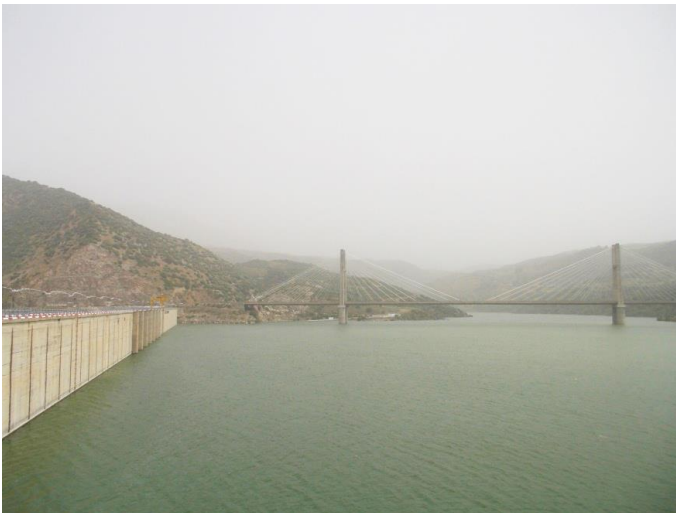
Photo 1: The largest dam in Algeria. The Beni Haroun dam with a capacity of 1 billion m 3 (Remini, 2014)
