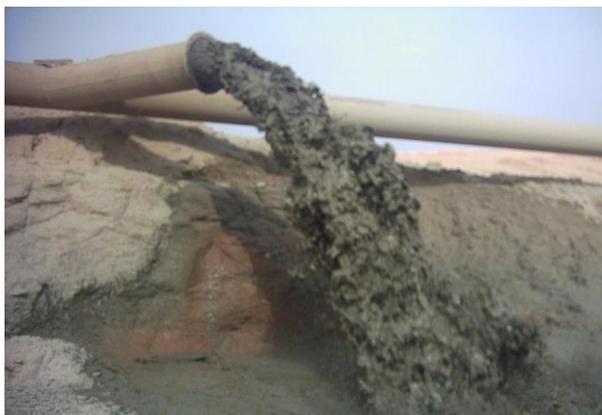
**Figure 5: Desilting of Foum El Gherza dam (Photo Remini, 2006)**
