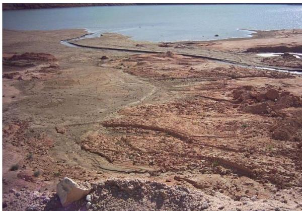
Figure 4: Progress of the sediment delta in the Foum El Gherza dam (Photo Remini, 2006)
