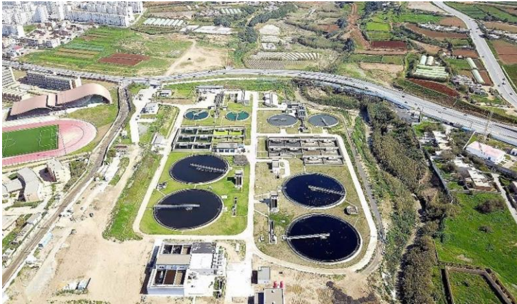
Figure 3: WWTP in the municipality of Beni Messous (Wilaya of Algiers) ( www.amenhyd.com )
