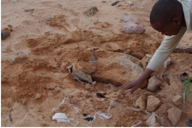
Figure 10: Foggara of Tafza: Operation of covering a kasria with flat rocks (Photo Remini, 2008)
