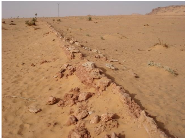
Figure 9: Seguia covered with rocks with a length of more than 200 m connecting the exit of the gallery to the main kasria of an Erg foggara of the Ouled Said oasis (Photo Remini, 2009).
