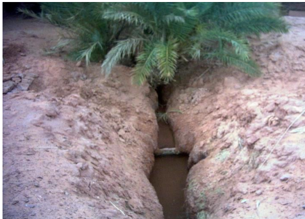
Figure 20: A view of the kasria from a Garden foggara in the central Timimoun palm grove (Photo. Remini, 2008)
