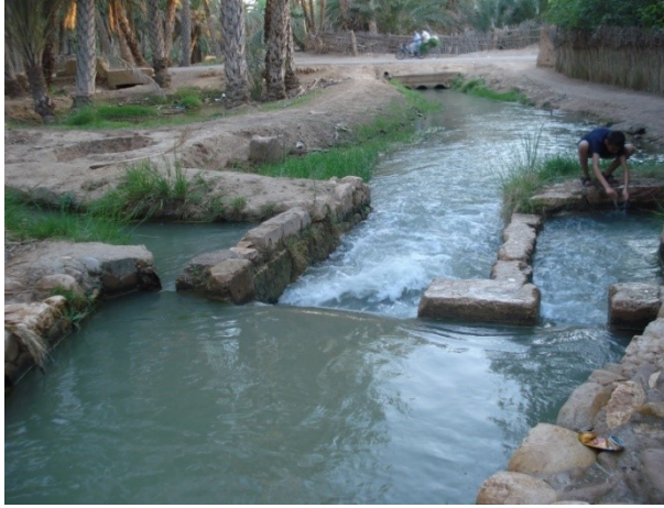
Figure 40: The large dam water distributor of Foum El Gherza in the oasis of Sidi Okba (Photo Remini, 2017)
