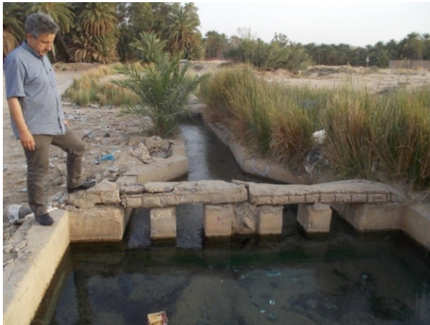
Figure 39: The main spring water distributor in the oasis of Chetma (Photo. Remini, 2017)
