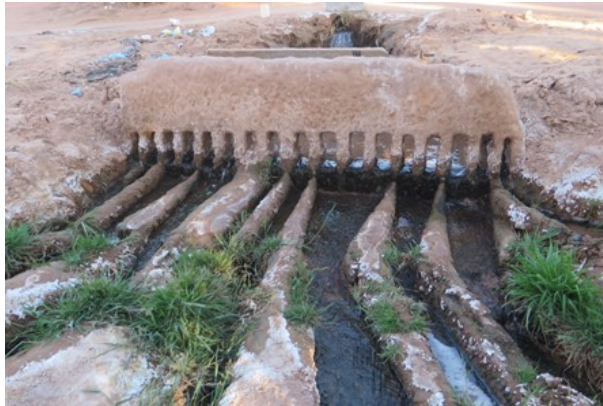
Figure 43: Secondary Kasria of the foggara of El Meghier in the Timimoun Oasis (Photo Remini, 2015)
