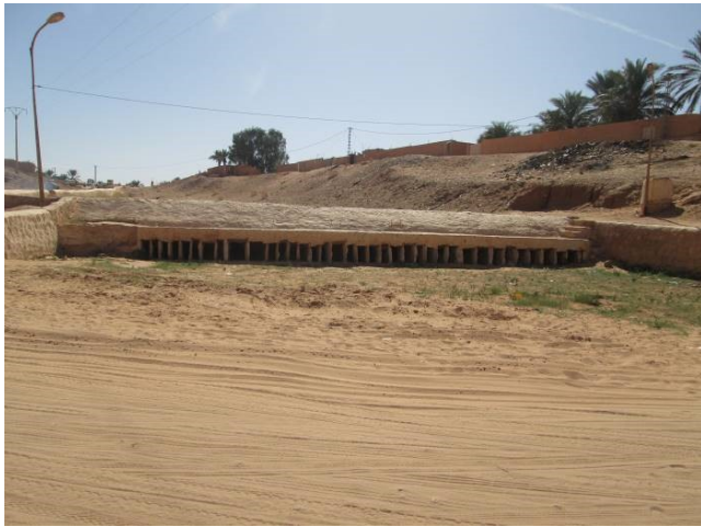
Figure 33: A general view of the Tissanbadh structure (Photo. Remini, 2014)
