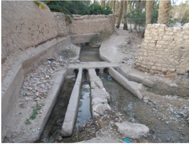
Figure 38: A secondary spring water distributor in the oasis of Chetma in the Ziban region (Photo. Remini, 2017)
