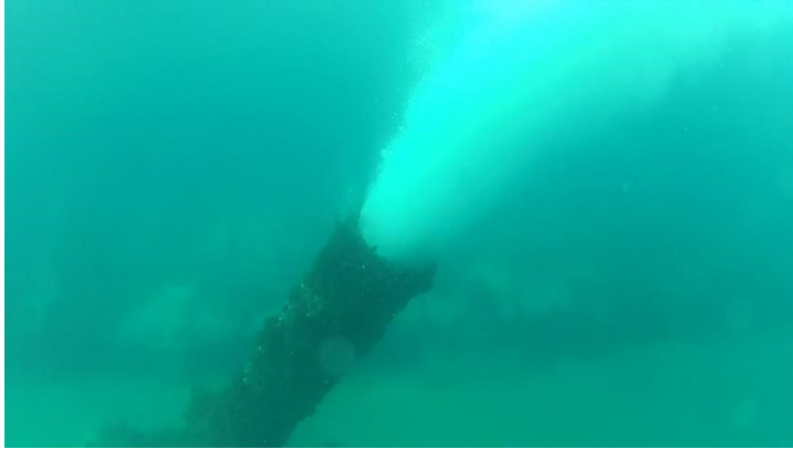
Figure 26: Direct discharge of brine to the seabed from a desalination plant in Algeria (Fouka Station)
