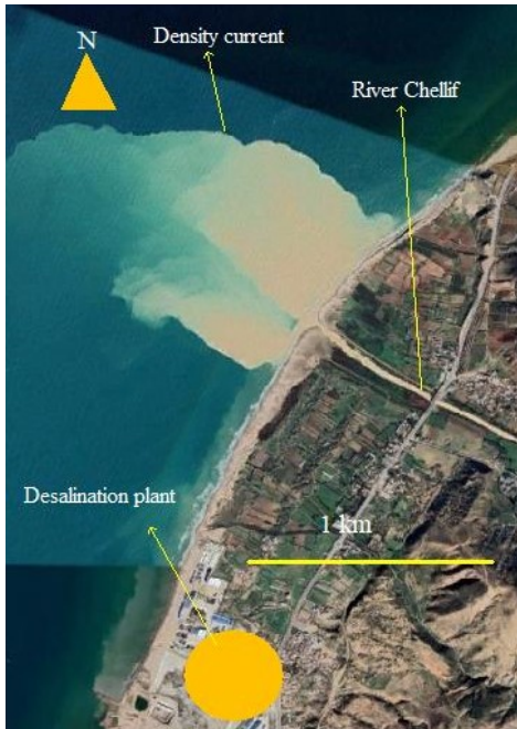
Figure 17: Formation of a density current during flood contact of the Chellif wadi with the sea (Google Earth)
